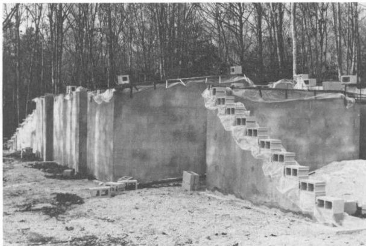
Fig. 2-10. David and Debbie Greenlaw are actually building above ground and then covering the home with earth.
