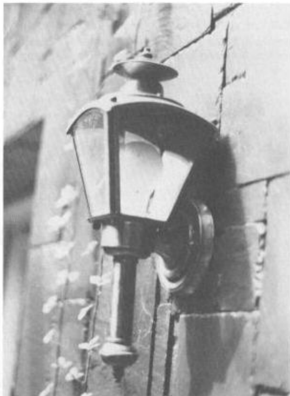
Fig. 16-12. Wall lighting is necessary.
