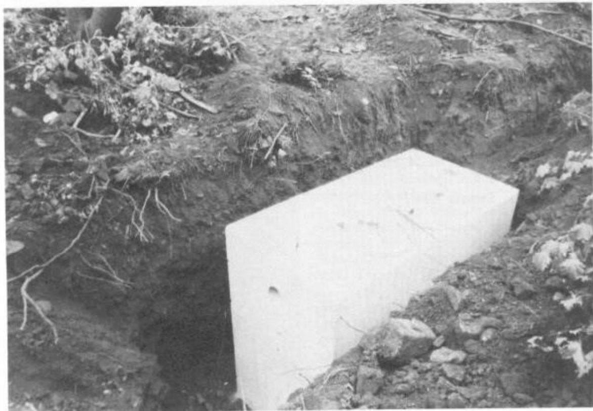
Fig. 6-7. Concrete septic tank in place.
