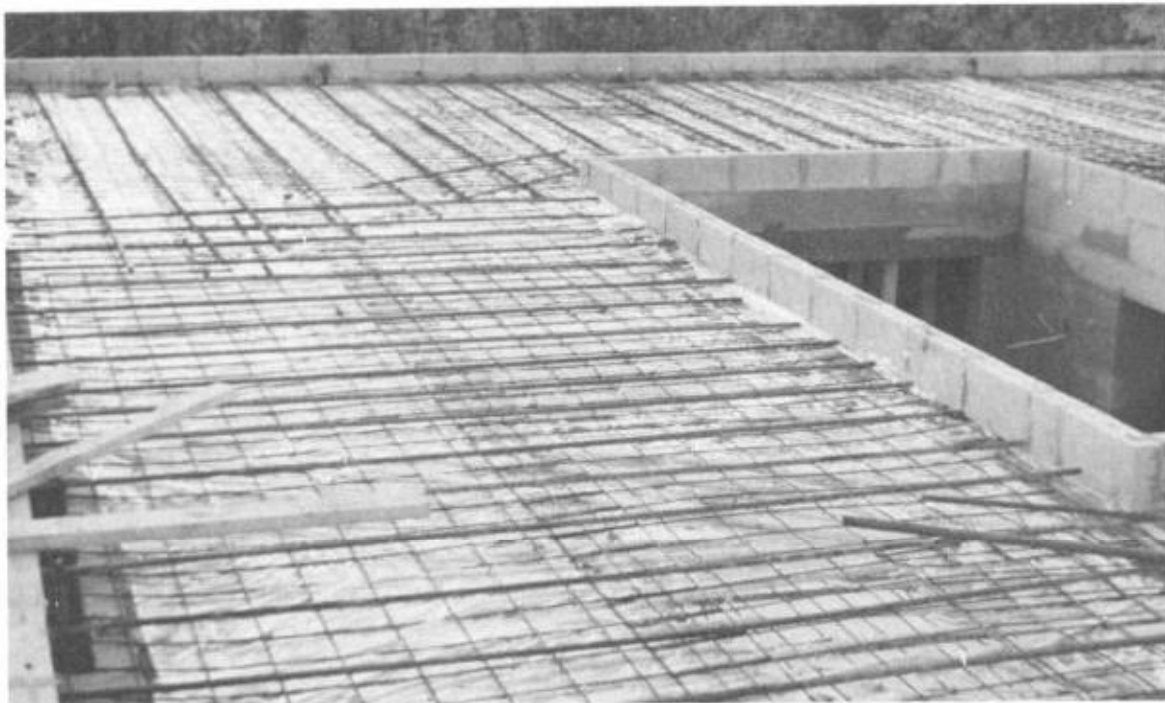
Fig. 9-17. Wire mesh gives real strength to the roof structure.
