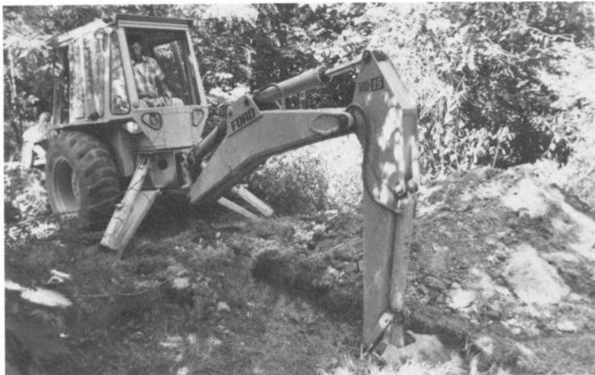
Fig. 4-5. A backhoe in the digging position.
