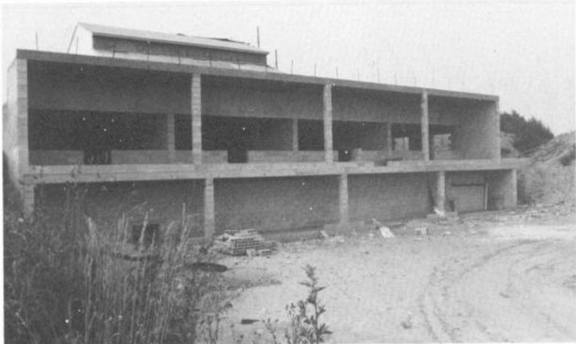
Fig. 10-10. One of the largest earth-sheltered homes in the country under construction.
