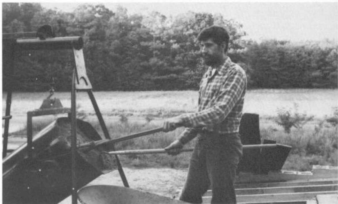
Fig. 10-6. Mr. Greenlaw using a home-made concrete mixer.
