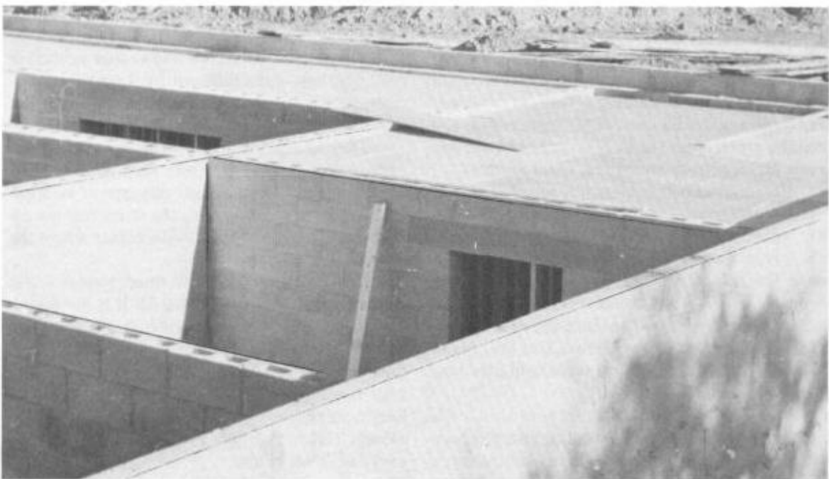
Fig. 9-2. This is how shoring looks once underway.
